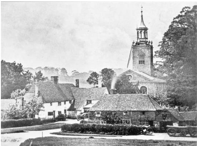
View to the west, from Stumble Hill, with the old inn – The Bull on the left and the smithy on the right – both demolished when the present church was built in 1881
